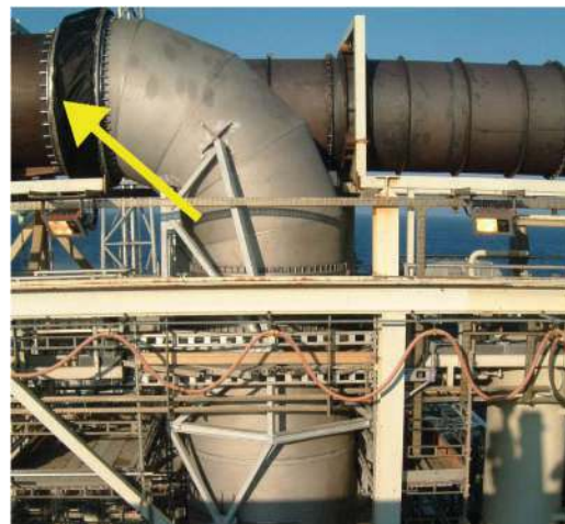
Thermobolt installed on an LM2500 Exhaust Duct.
